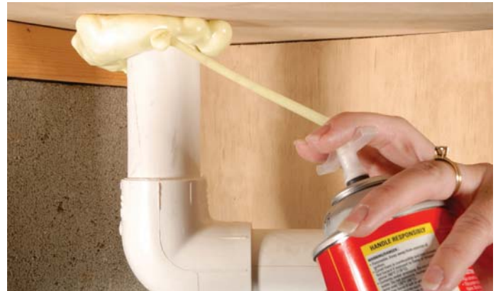
Many homes lack adequate insulation or have gaps that need air sealing.
